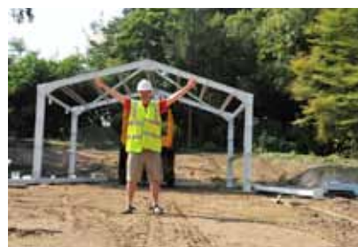
David in front of the steel work
