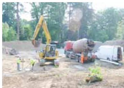
Foundations for joinery workshop
